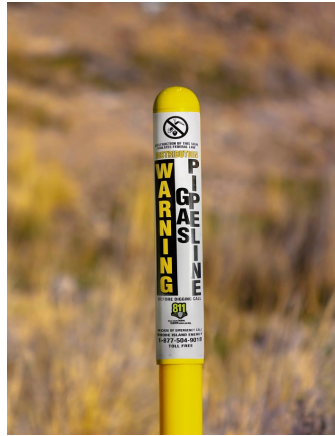
Rhode Island Energy pipeline marker.
