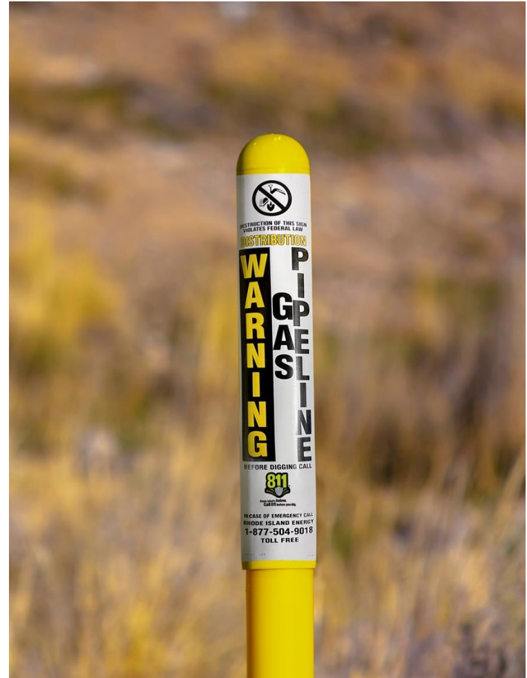
Rhode Island Energy pipeline marker.
