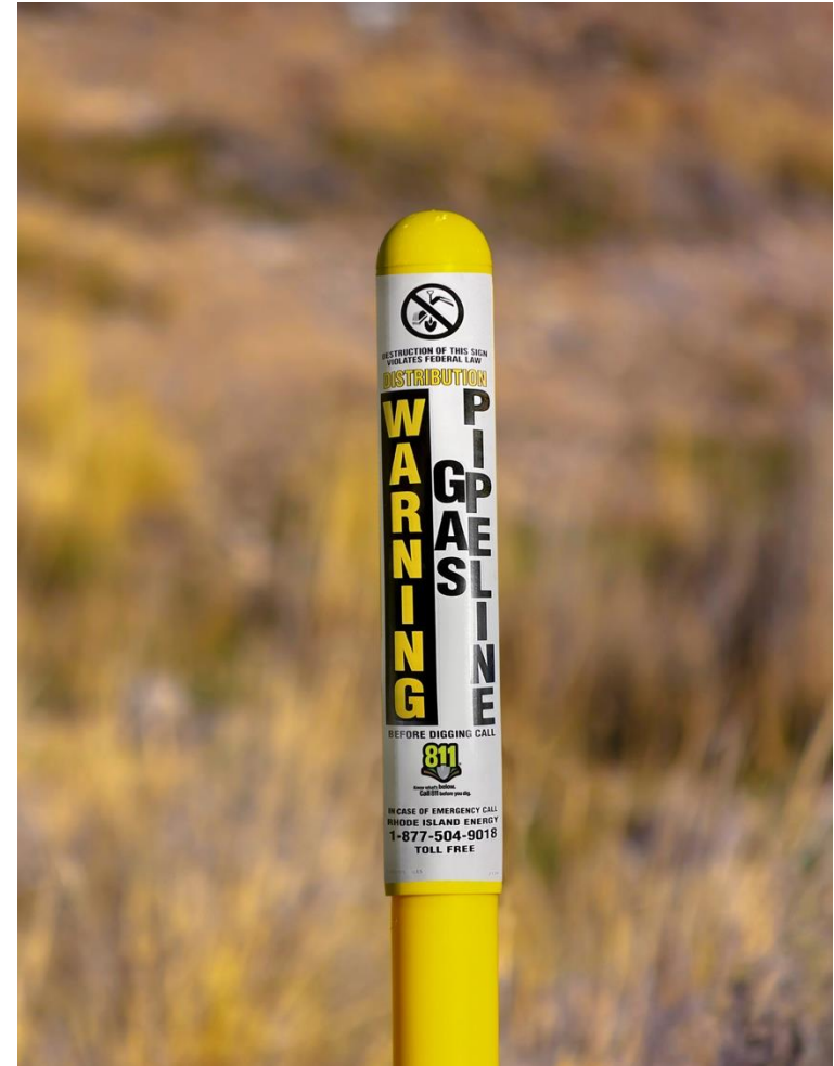
Rhode Island Energy pipeline marker.
